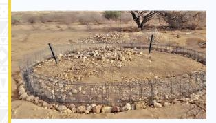
A 200-meter-long pipeline, installed with support from the Danish International Development Agency (Danida) and NRT's Water Program, draws water straight from the Ewaso Nyiro River and temporarily stores it in a 30 cubic meter concrete tank for 12 hours, where silt and other waste are filtered out.
